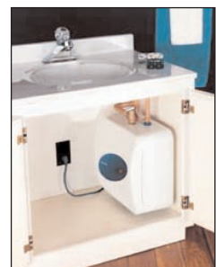
Figure 4: A typical electric demand type boiler.
